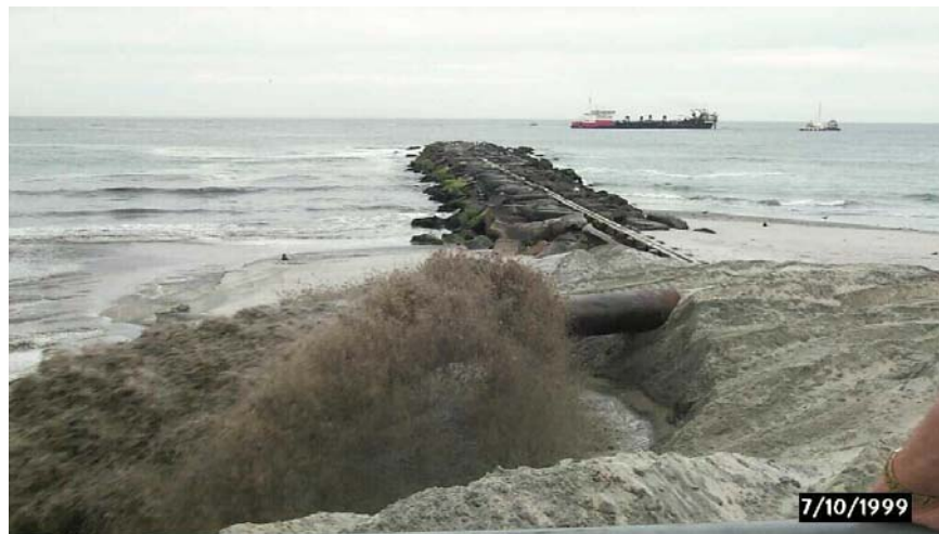
Figure VI- 2: Beach fill operation with discharge from pipe.
