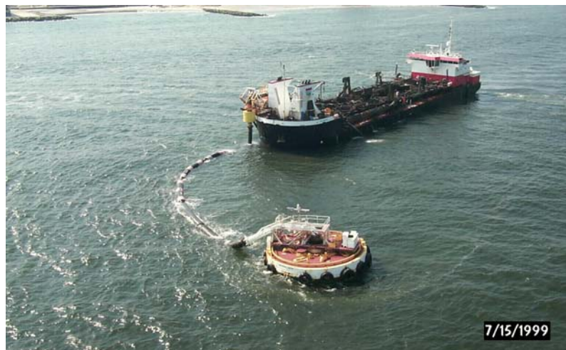
Figure VI-1. Dredging at an offshore borrow site.
